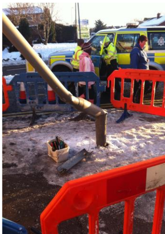
Damaged in RTA
